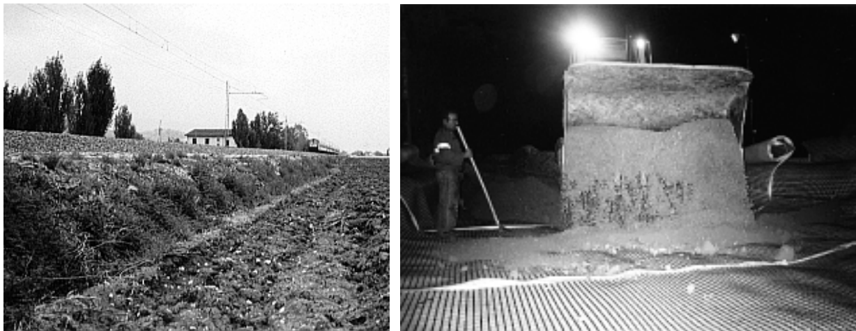
Figure 4: Reconstructed railway line and geocomposites fill covering during the night.
