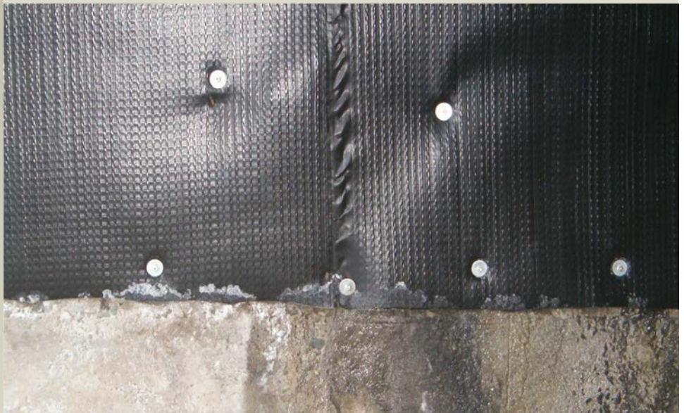
Photograph showing the supporting anchors holding the drainage liner.
