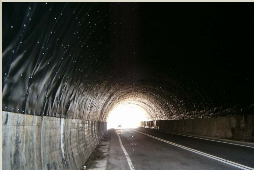
Installed Tenax Drainage Lining system at Palmentello tunnel, Italy.
