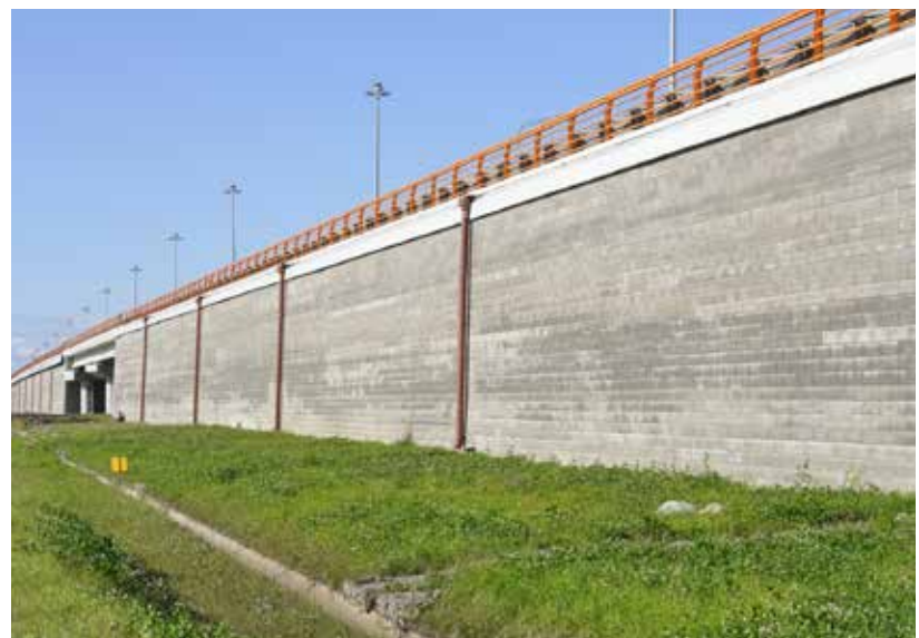
St. Petersburg ringroad, Russia: Geogrid reinforced wing wall.
