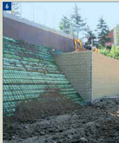
Photo 1: Built with green slope. Photo 2: Curved walls. Photo 3: Built with ramp. Photo 4: Built with fence. Photo 5: Built with steps. Photo 6: Built with reinforced slopes. Photo 7: Built with concrete structure.
