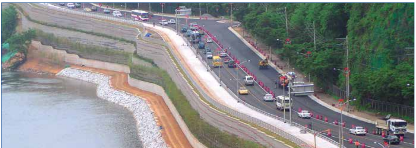
Chunsugyo, South Korea Saebeari Highway: Geoblock segmental retaining wall System.
