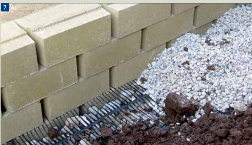
Photo 1: Foundation with curb.
