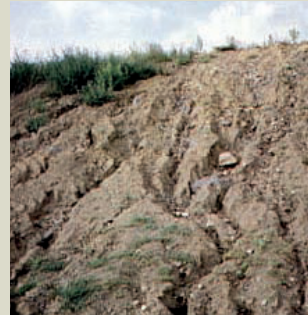
Figure 1: Natural development of water rills on embankments
