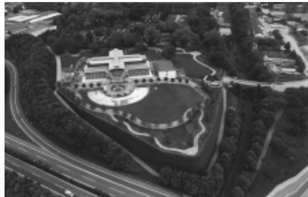
Figure 13: The whole construction
