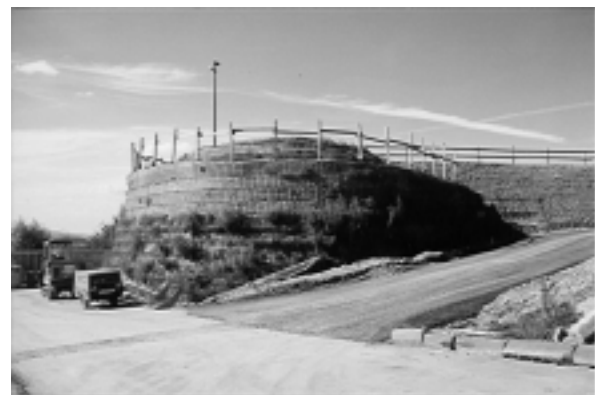
Figure 9: Circular building at the south end of the construction
