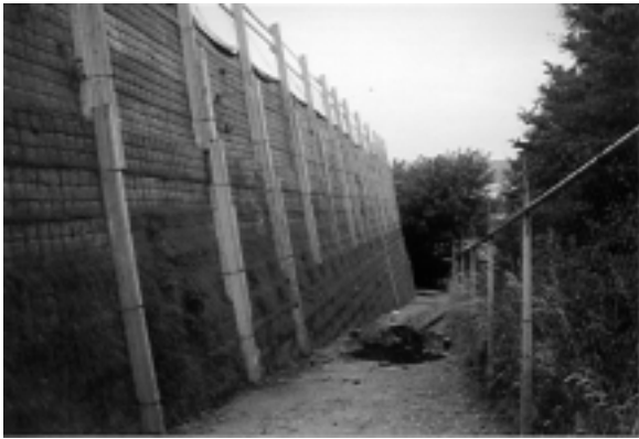
Figure 6: North side of the construction during building
