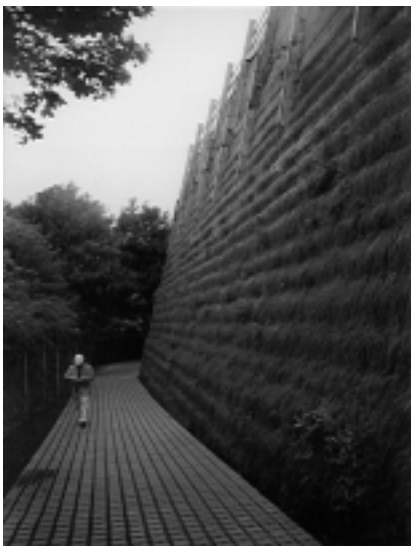
Figure 8: West surface during construction, half complete
