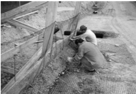
Figure 7: Installation of a wedge of topsoil
