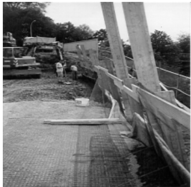
Figure 3: Detail of work on the facing
