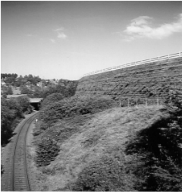
Figure 10: West side, completed
