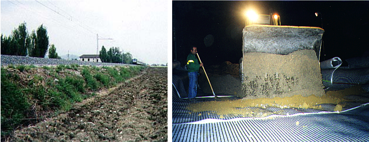
Fig. 2 Reconstructed railway line and geocomposite fill covering during the night
